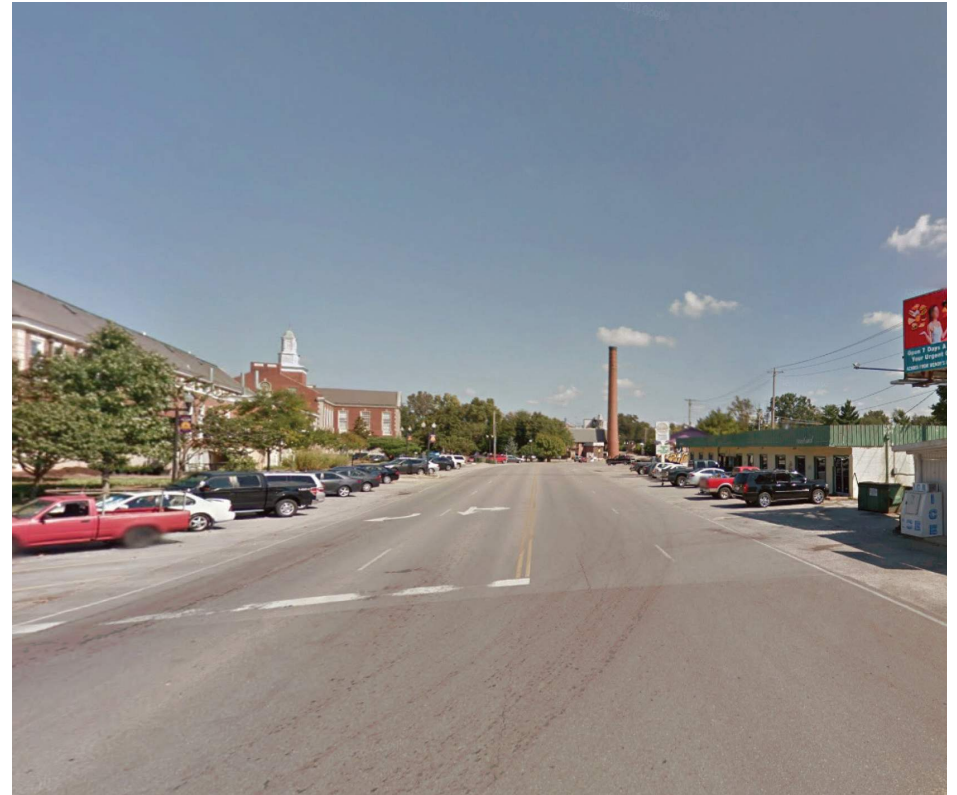
Figure 2.15 Mahler Avenue, north of West 7th Street
