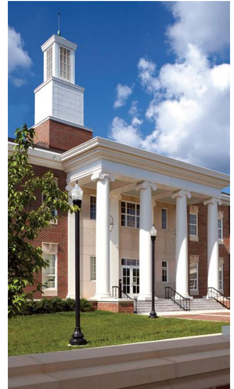
Figure 3.8 Bell Hall courtyard
